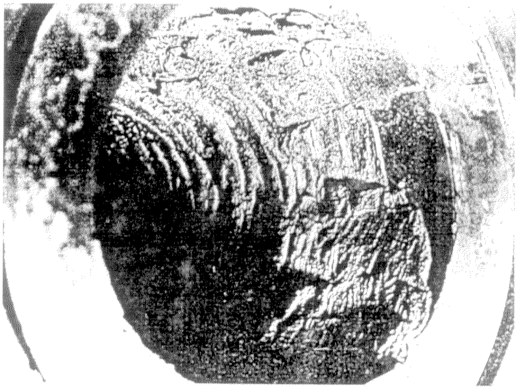
Pipe condition before lead-bismuth technology improvement program
